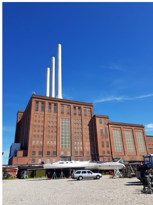
Orsted's Svanemølle District Heating Power Station, Copenhagen. Source: 4D Infrastructure
