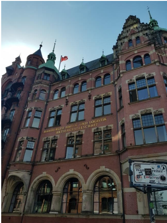
Hamburger Hafen Head Office, Hamburg. Source: 4D Infrastructure
